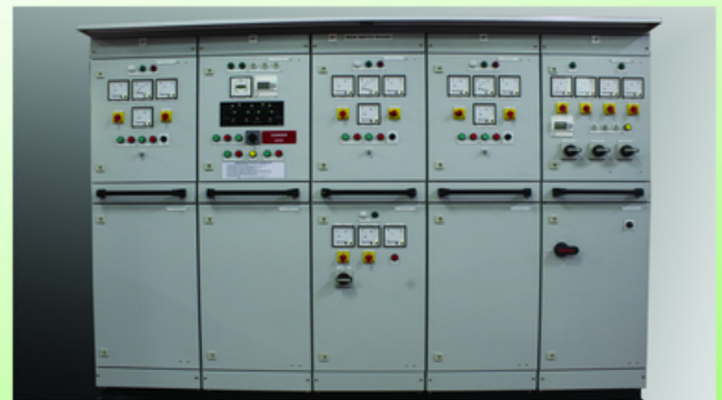
MSB for Floating Border Out Post (FBOP) Vessels Certified by IRS for BSF
