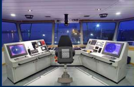
Wheel house AFT Console for Anchor Handling Tug Supply Vessel
